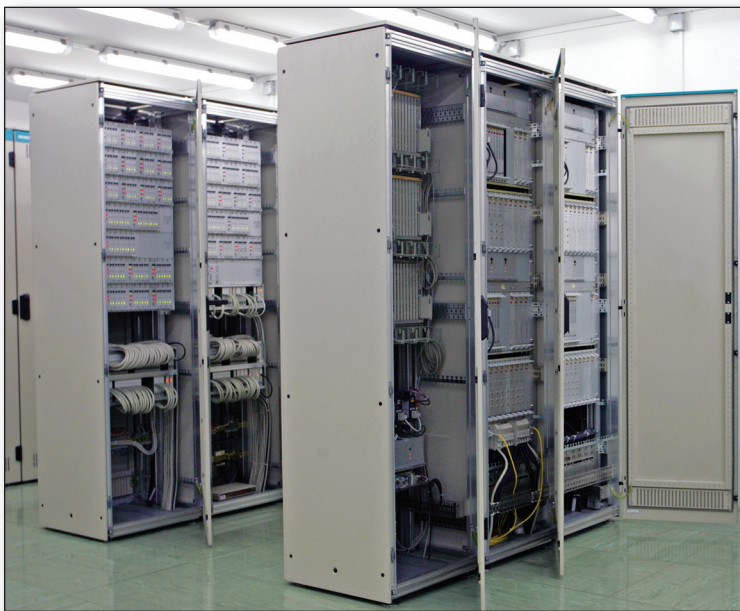
Figure 3. Railway Interlocking System Hardware.
