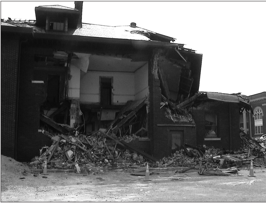
Figure 1. Lebanon Town Library Partially Demolished under INTF-1's Direction to Simulate an Earthquake.
